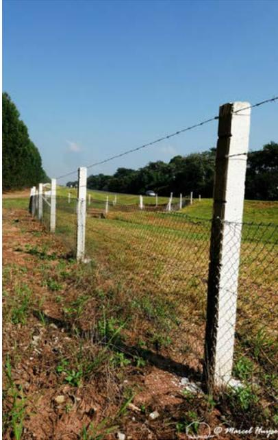
**Figure 4: “Wildlife” fence that is basically a livestock fence with chain-link attached to the lower portions of the fence posts, along SP-225, near Brotas, São Paulo, Brazil (© Marcel Huijser).**
