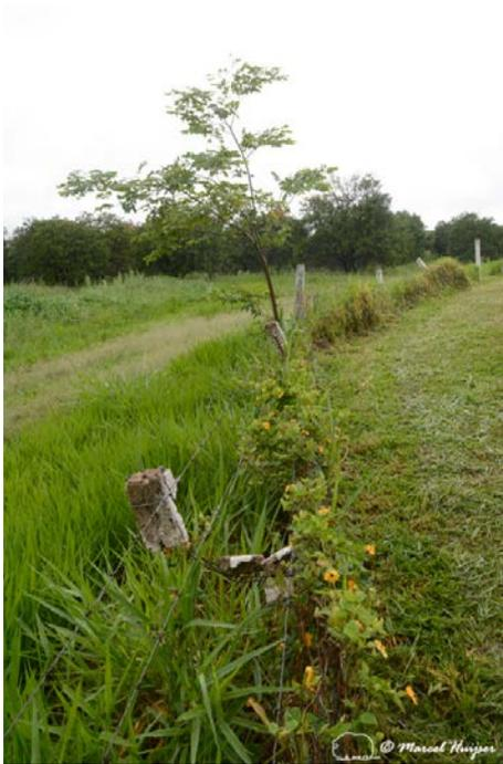
**Figure 7: Disintegrated fence posts of a “wildlife fence” overgrown with vines (i.e. this is essentially a livestock fence with chain-link attached to the lower portions of the fence posts), along SP-225, near Brotas, São Paulo, Brazil (© Marcel Huijser).**
