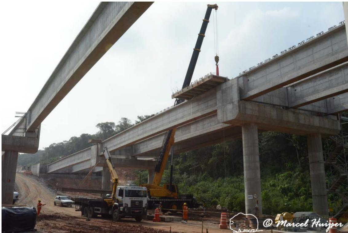
**Figure 19: Overspan bridge under construction, Rodoanel Norte, São Paulo, Brazil (© Marcel Huijser). Note that the vegetation has been removed, and that the soil has been compacted everywhere by heavy machines.**
