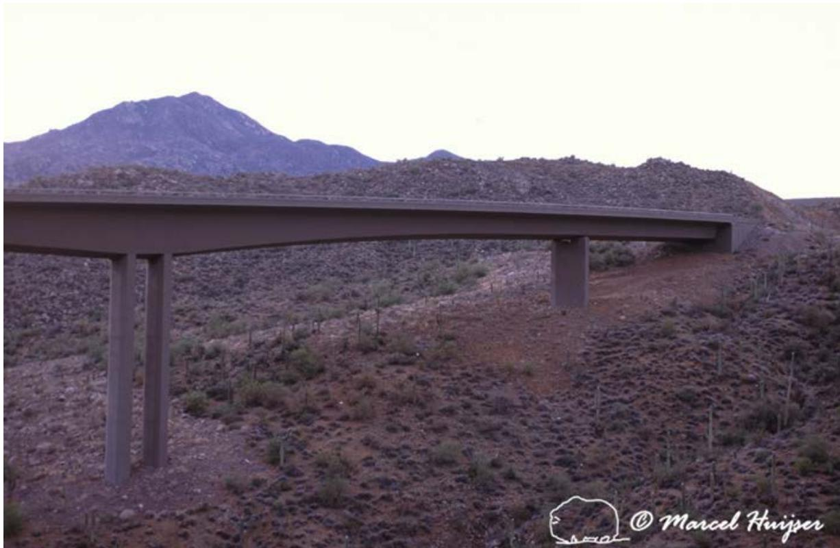
**Figure 20: Overspan bridge shortly after construction, Tonto National Forest, Arizona, USA (© Marcel Huijser). Note that the impacts of the construction on the vegetation and soil have been minimized.**
