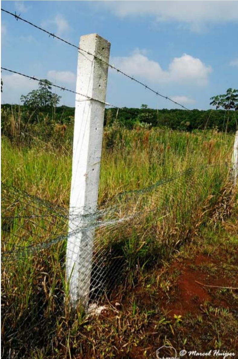
**Figure 6: Damaged “wildlife fence” (i.e. this is essentially a livestock fence with chain-link attached to the lower portions of the fence posts), along SP-225, near Brotas, São Paulo, Brazil (© Marcel Huijser).**
