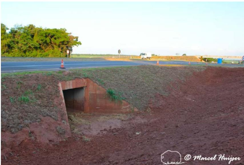
**Figure 15: Wildlife underpass (concrete box culvert), along SP-270, about 70 km south east from Presidente Prudente, São Paulo, Brazil (© Marcel Huijser). There is an uphill slope towards the right of the image. It would be better to have a level approach for wildlife when they approach the structure (no slope).**
