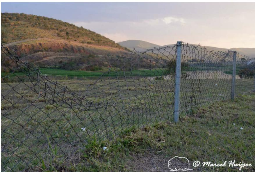
**Figure 8: Damaged “capybara fence” (though this fence is much too low to be an effective barrier for capybara), along Rodovia Presidente Dutra (BR-116 – SP-60), near Lavrinhas, São Paulo, Brazil (© Marcel Huijser). Note the bare spots in the vegetation on either side of the fence indicating that wildlife, presumably capybara regularly jump the fence at this location.**
