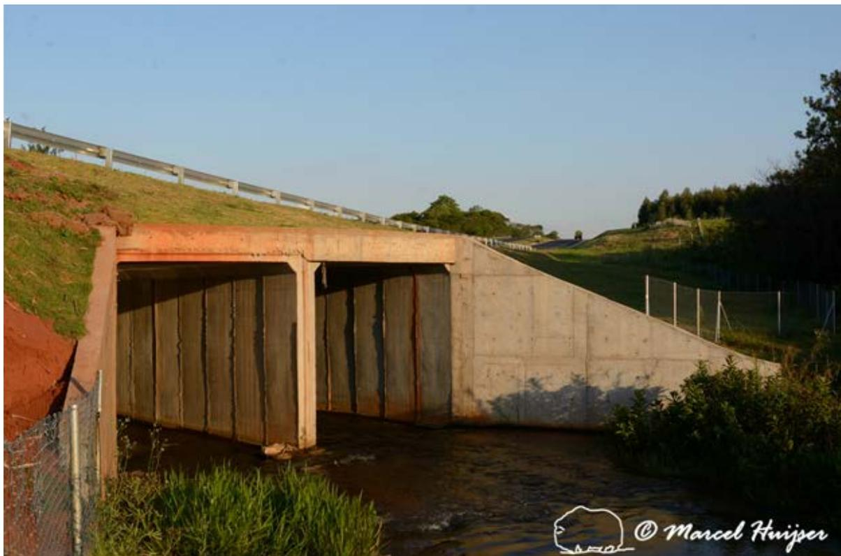
**Figure 18: Multi-functional underpass (water, wildlife) with a dividing wall (the structure basically consists of two box culverts), along SP-270, about 70 km south east from Presidente Prudente, São Paulo, Brazil (© Marcel Huijser).**
