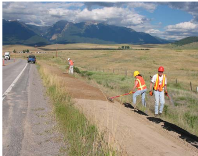
Figure 9: Raking the sand material to evenly cover the track bed fabric.
