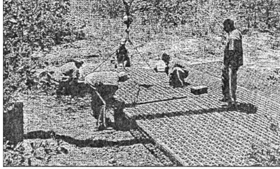
Figure C-19: Installation of deer (bridge) grate used in deterrence tests for Key Deer, Big Pine Key, FL 2001-2002 (Peterson et al. 2003).
