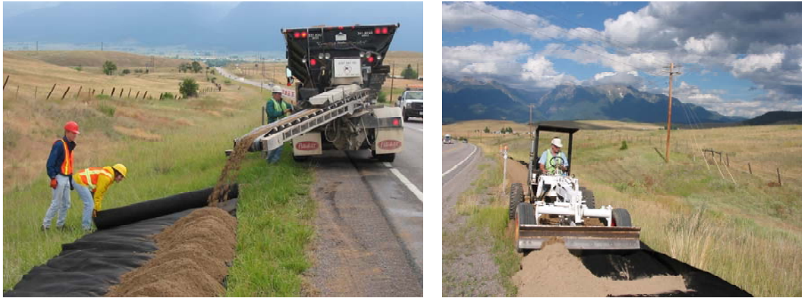
Figure 8: Rolling filter fabric out while sand material is distributed by a conveyor belt (left) and spreading the sand with a grader (right).
