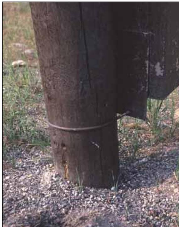
Figure 8.4: The problem with some of the break-away constructions for the wooden poles was addressed by drilling new holes at the appropriate height above the ground level. (Photo: Marcel Huijser, WTI-MSU)
