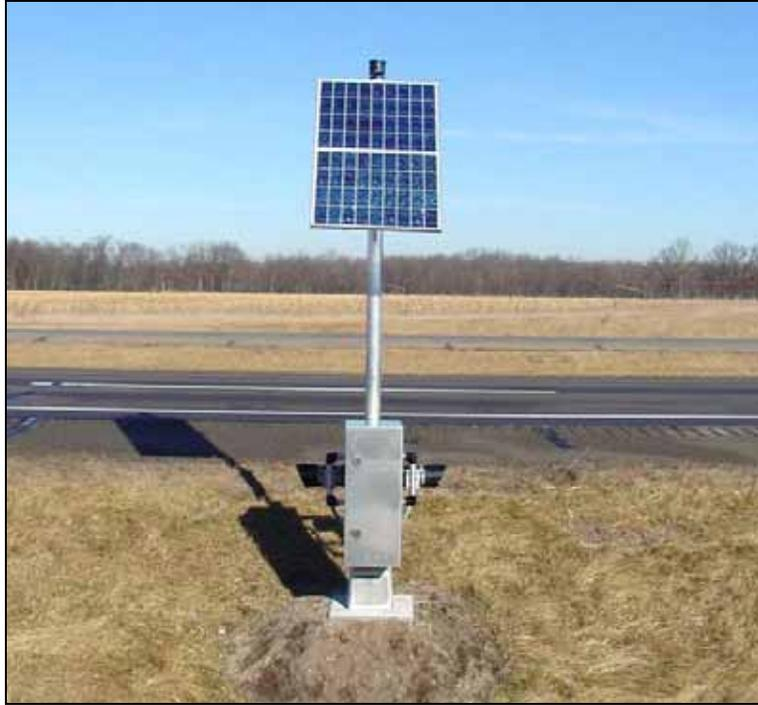
Figure 4.32: Pole with sensor tubes, cabinet (with circuit boards and batteries) and solar panel on the Indiana Toll Road, Indiana, USA (Photo: Indiana Department of Transportation, Toll Road District)
