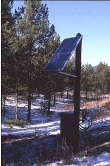
Figure 8.7: Care should be taken that solar panels are not placed in the shade of trees or other objects, including steep slopes. The angles of the sun should be calculated during winter, as daylight is scarce and the sun is low on the horizon. (Photo: Marcel Huijser, WTI-MSU)
