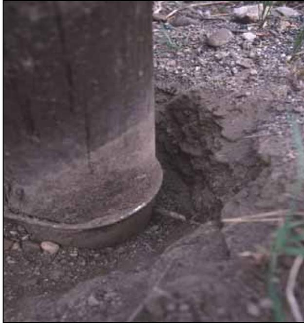
Figure 8.3: Some of the wooden poles were buried too deep. The stick indicates the upper of the three holes that serve as a break-away in case of a collision. All three holes should have been above the ground level. (Photo: Marcel Huijser, WTI-MSU)
