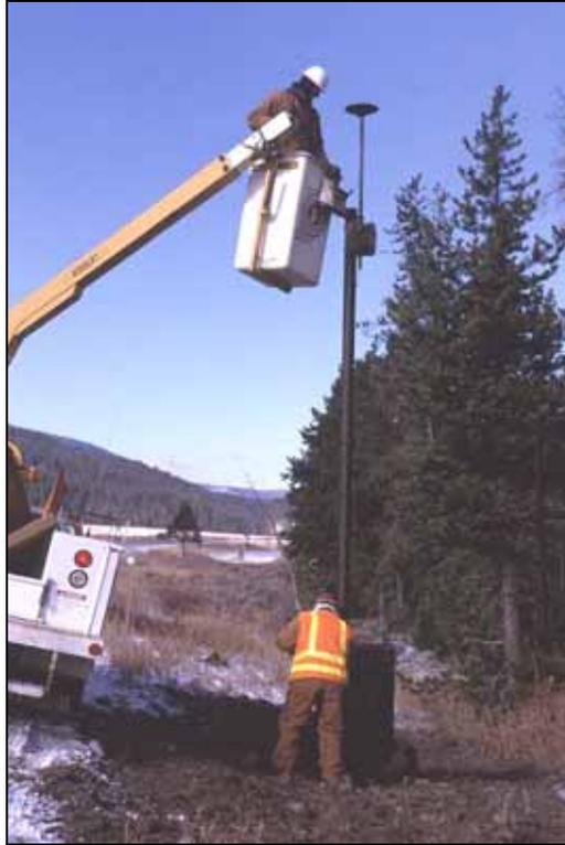
Figure 5.23: Installation of the antennas, beacons, signs and solar panels at the MT site required the use of a bucket truck (Photo: Marcel Huijser, WTI-MSU)
